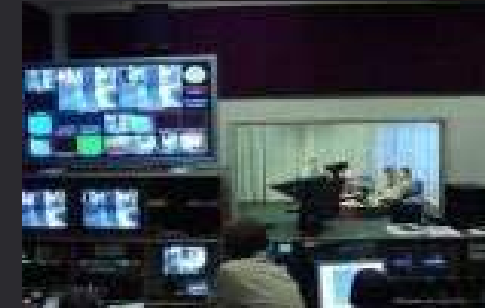
MPC-H Control Room
